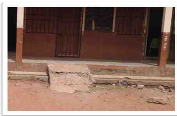
Figure 26. Defective ramp
