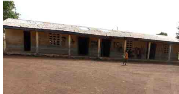
Figure 25. Classrooms with no ramp
